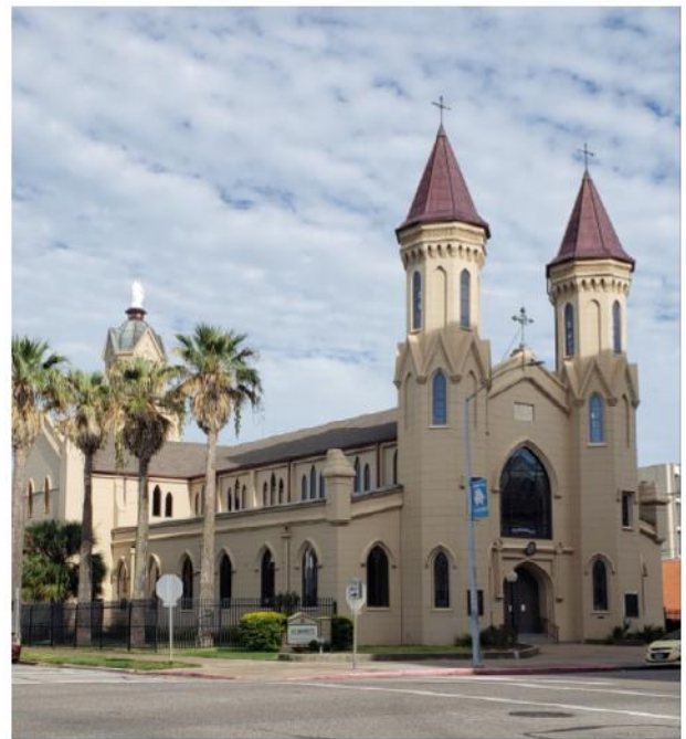
St. Mary's Cathedral Basilica 2011 Church Street, Galveston, TX
